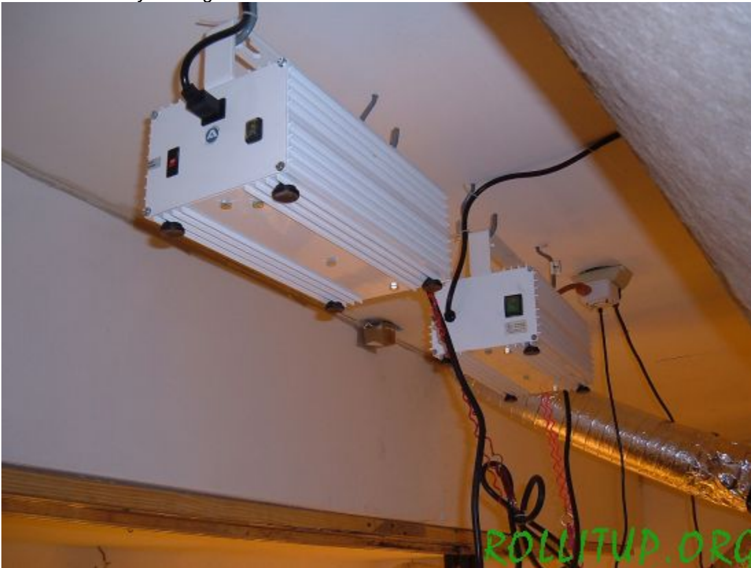
The ballast for my HPS lights.
